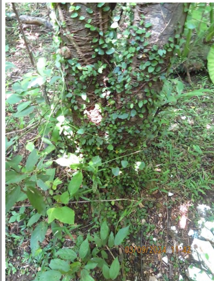
Root flare condition
